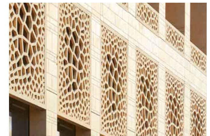
this page: Wall screens, roof screens, and façade textures contribute to the placemaking aspects of a new Qatari architecture. These elements are designed by John McAslan + Partners (left) and Gensler (top and above).
